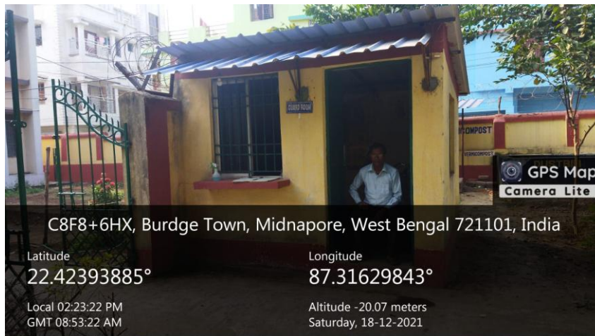
Guard Room of Women's Hostel
